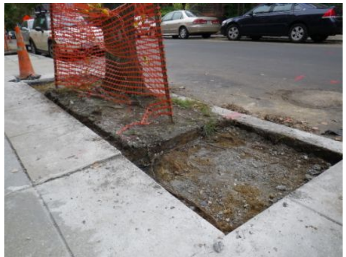
Kalorama Rd tree-box after concrete removal. Photo: Ted Guthrie
