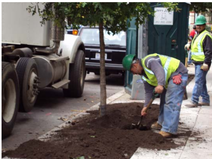
Workers spread topsoil in an expanded tree-box on the 1800 block of Kalorama Road. Photo: Steve Mckindley-Ward
