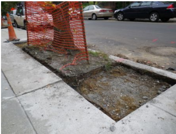
Kalorama Rd tree-box after concrete removal. Photo: Ted Guthrie
